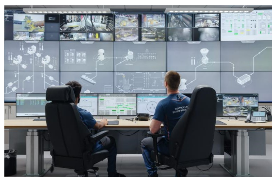
Figure 2.10: Elkem's Control Room in Breanger (Afry, 2023)
