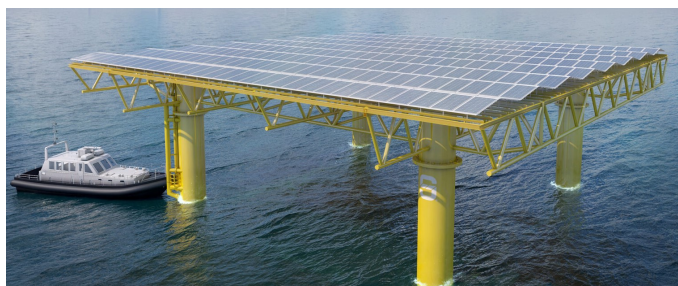
Figure 1.1: An offshore elevated floating PV system installed at the Port of Ostend, in the North Sea coast of Belgium [13].
