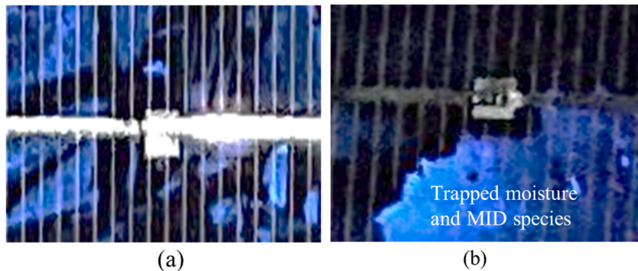
Fig. 4. Part of a solar cell and degraded copper ribbon showing signs of moisture ingress. Images were acquired under (a) clear sky outdoor and (b) optimized light exposure dark room conditions from the same area of the solar cell.
