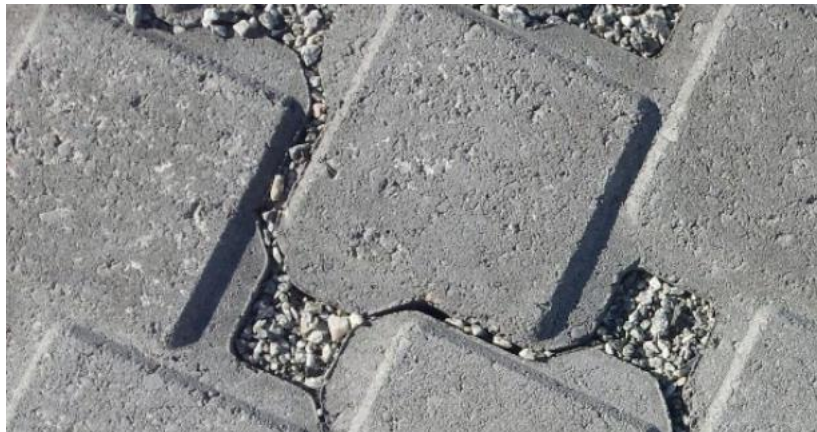
Fig. 3.16 – Permeable dekker [52]
