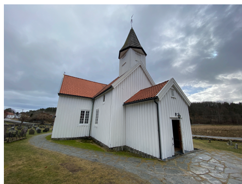
(b) Exterior View from West
