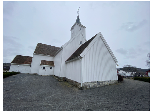
(b) Exterior View from West
