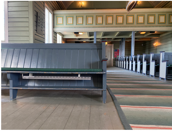
(a) Pew-mounted Bench Heater, 250W
