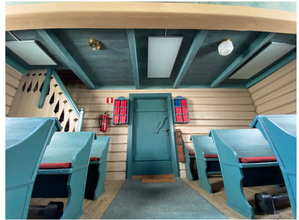
(b) Ceiling-mounted Heating Panels
