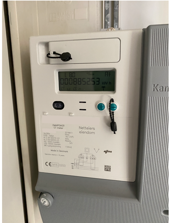
Figure 3.10: Smart Energy Meter (AMS)
