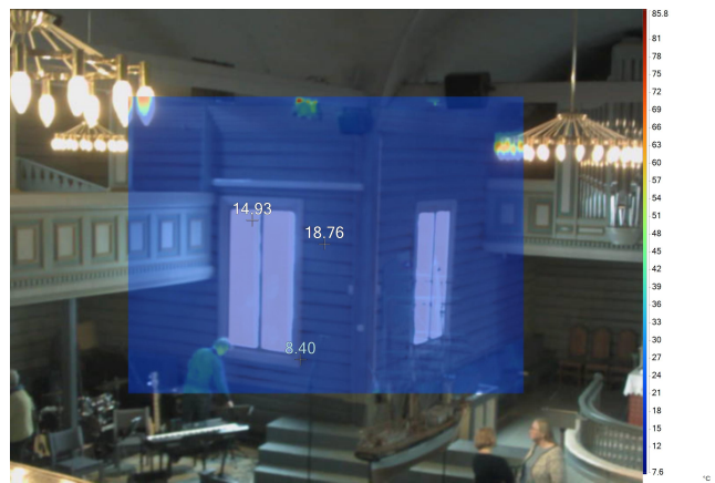
(a) Heat Loss around Window Frame
