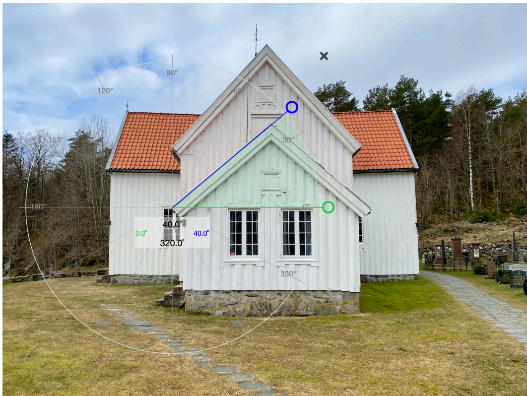
Figure 3.19: Roof Angle Measurement Eide Church
