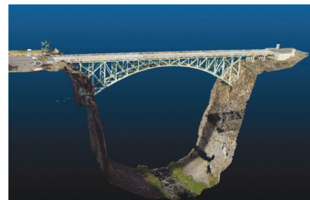
FIGURE 9: 3D point cloud of the crooked river bridge [91].
