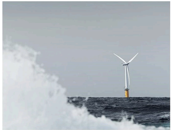
Fig. 1. Image of Hywind Demo, the world's first megawatt-sized floating wind turbine, located 10 km off the west coast of Norway. Source: Equinor ASA.
