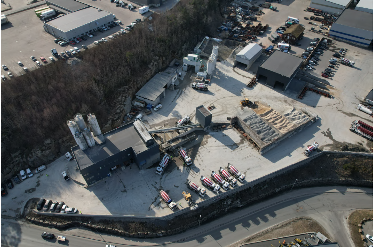
Figure 5.2: Overview of Ribe Betongs production line in Kristiansand. Foto: A. Verma [107]
