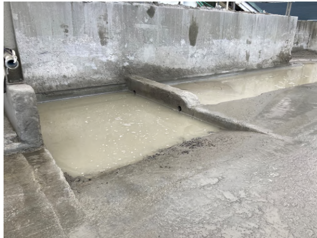
Figure 3.5: Sedimentation basins for concrete slurry and washing water
