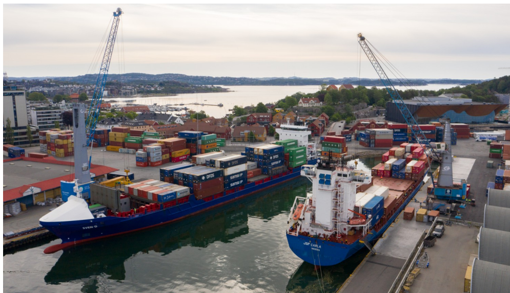
Figure 4.2: An Overview of the U-shaped Quay at Lagmannsholmen (Port of Kristiansand, n.d.-a)
