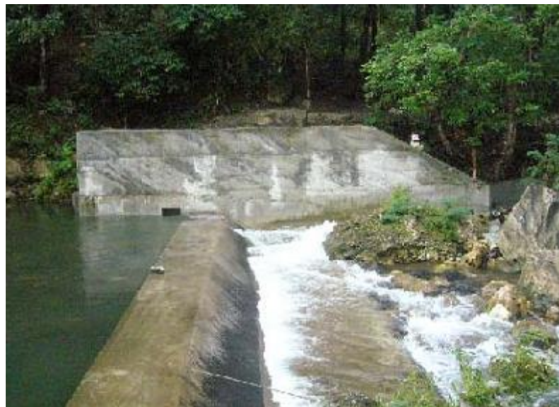
Figure 3.10 : Diversion Weir and Intake [32]
