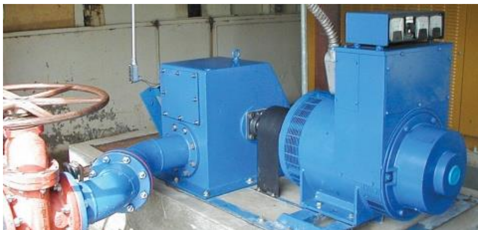
Figure 3.15 : Connection arrangement between Turbine and Generator [32].
