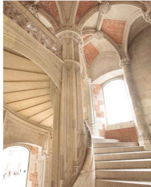
Figure 3.23 – Northern staircase of the Louis XII wing, Blois, France (1501) [47].
