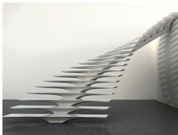
Figure 3.25 – Modular Pre-stressed UHPC Staircase (2009) [49].
