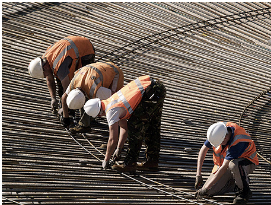
Figure 2.2 – Steel fixers [11].
