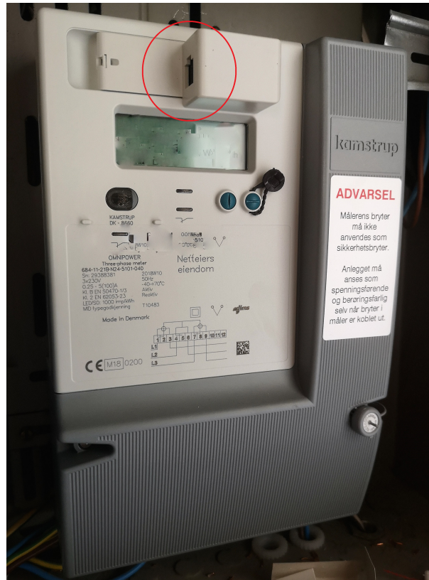
Figure 7: The HAN-port market with a red circle on an AMS from Kamstrup .
