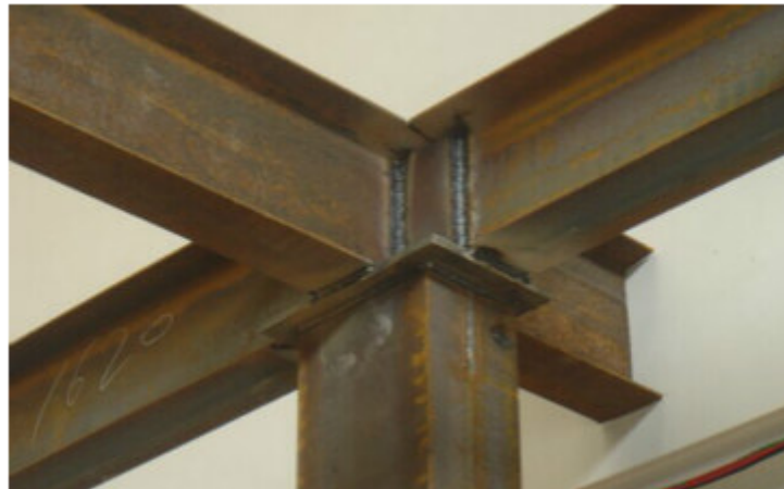
Figur 3.17: Welded connection[9]
