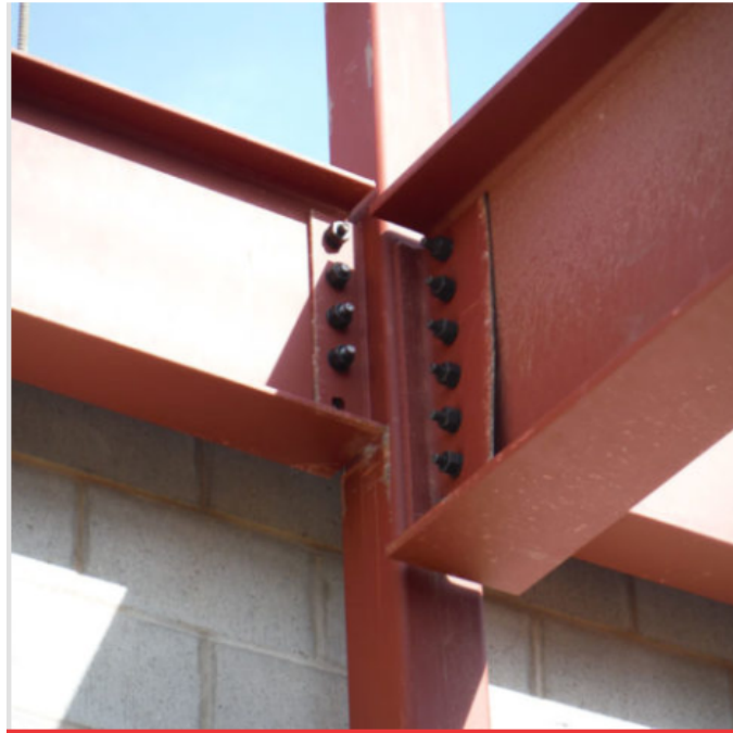
Figur 3.15: Bolted connection[8]
