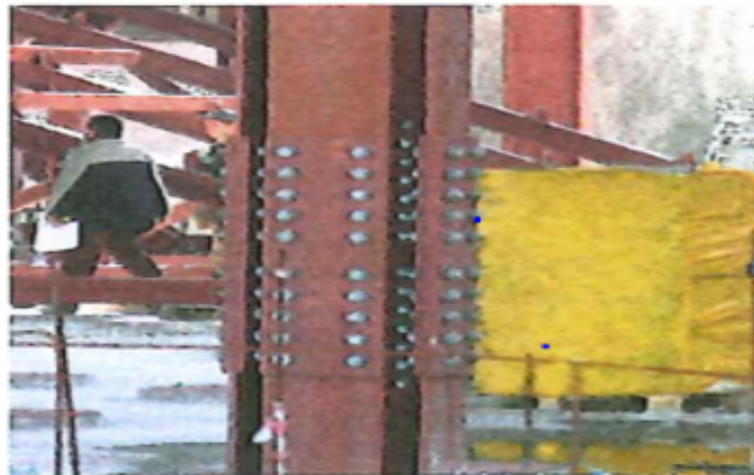
Figur 3.5: Continuity of column with double cross I-section [3]
