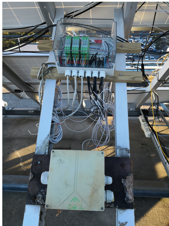
Figure 17: Shows the new transparent IP67 box compared to the old one
