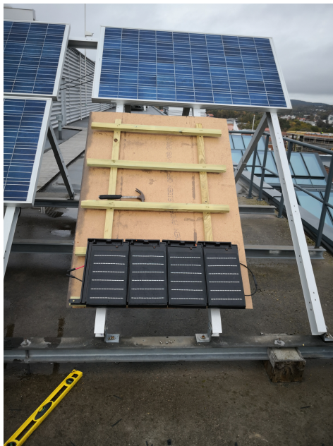
(a) Demo roof with only one row of roof tiles
