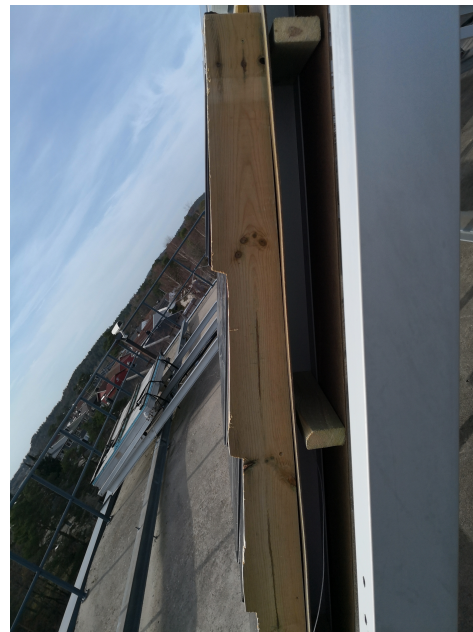
(b) Cold attic room
