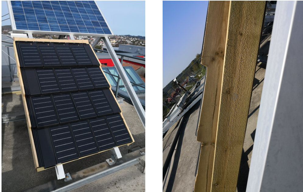
(a) Shows the demo roof
