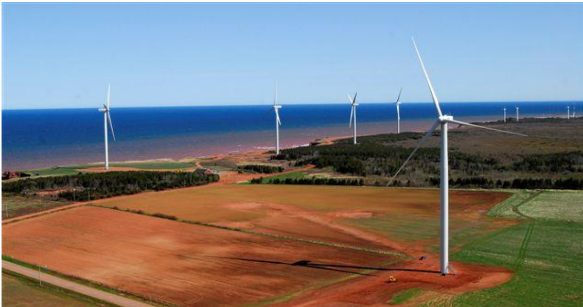
Figure 15. WEICAN 10 MW wind farm. From (Canada, 2018)
