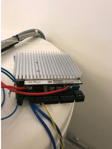
Figure 31 Picture of the Thyro after it is installed.
