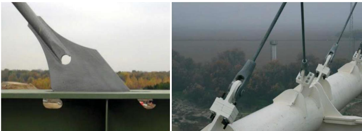
Figure 3.11: Left: Welded connection for steel rod, right: fork connection for spiral strand cable [16].
