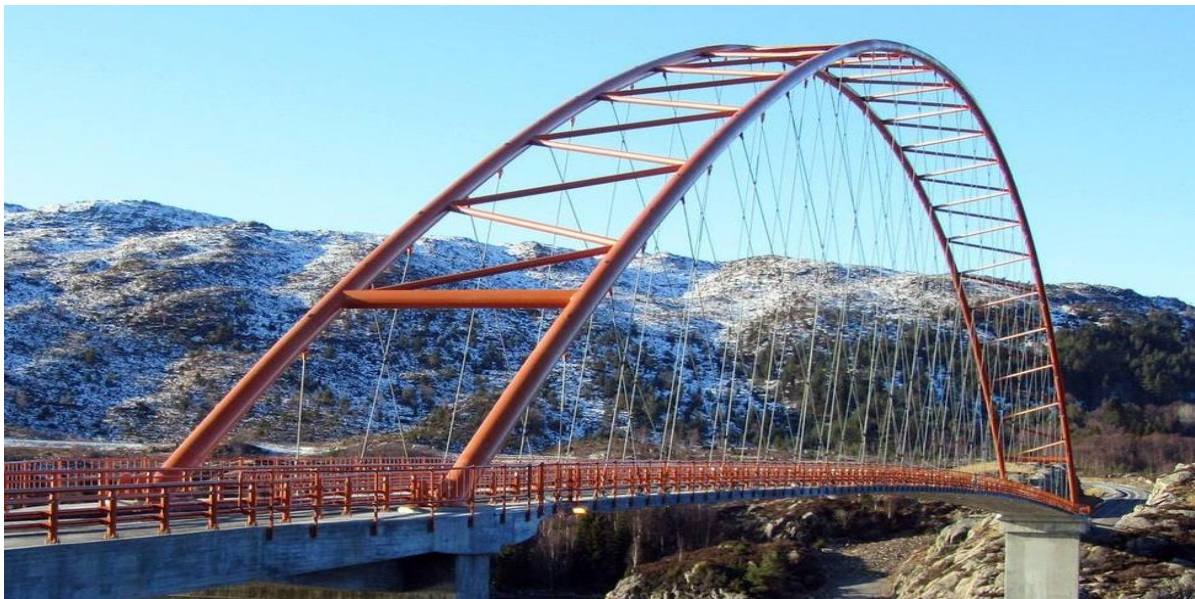
Figure 3.4: Brandangersundbrua with circular hollow arches [9].
