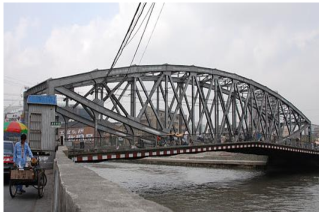
Figure 3.2: Da Vinci's drawing, right: Lenticular girder in Shanghai [4].
