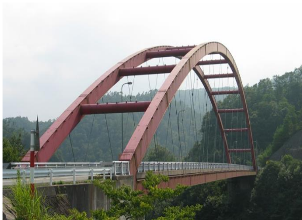
Figure 3.5: Tsukani Bridge with box-section arches [10].
