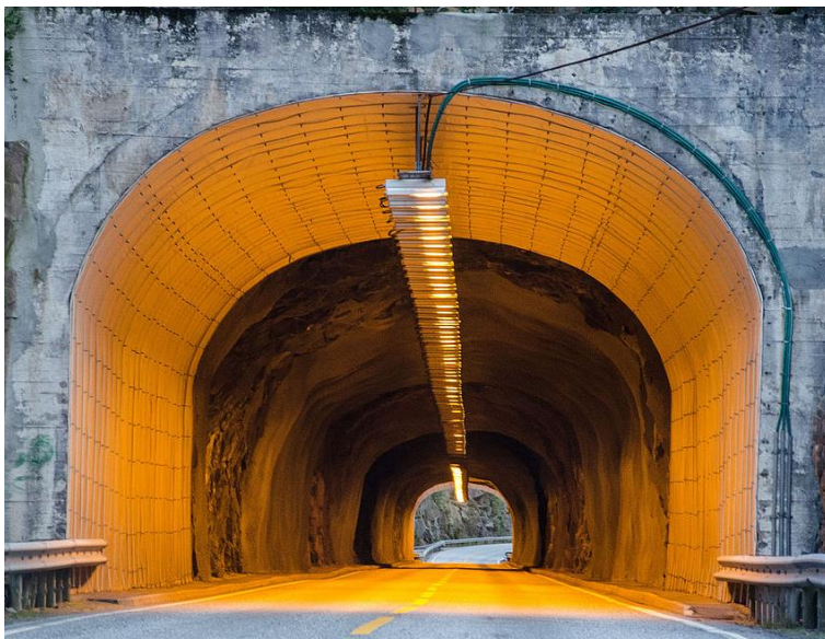
Figure 8-2 Photo of a rock tunnel, Trøde-Bråhei in Lillesand [7]
