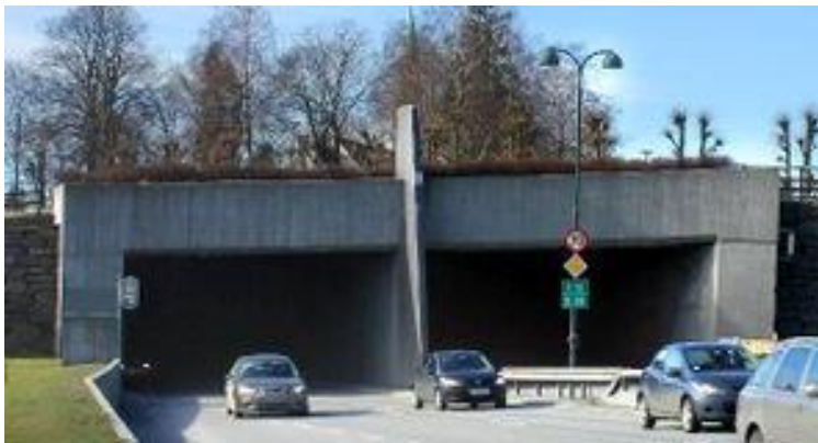
Figure 8-1 Photo of a load-bearing concrete tunnel, Oddernestunnelen in Kristiansand [6]
