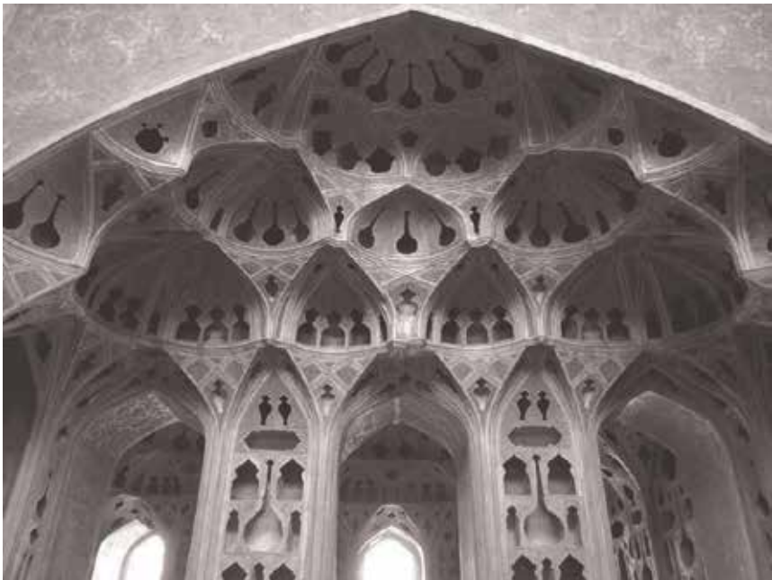
Figure 4.10. Music Room. The acoustic ceiling of the rooftop music room of the Ali Qapu Palace in Isfahan, Iran. Photo: David Stanley. Published on Flickr under a Creative Commons Attribution 2.0 Generic license (CC BY 2.0); some rights reserved. Original photograph in colour.
