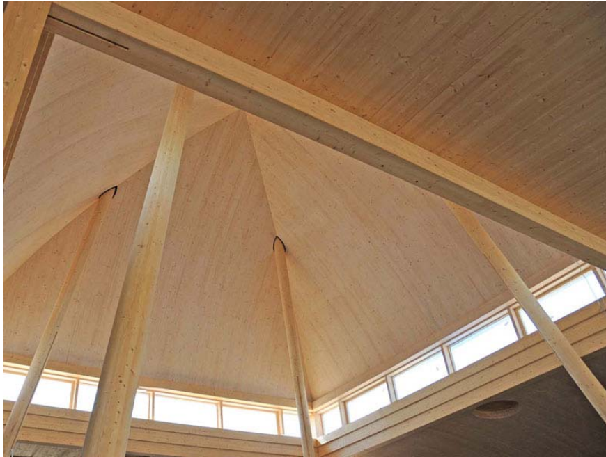
Figure 5.21: Example of a CLT-construction: evangelic church in Regensburg, Germany [5]
