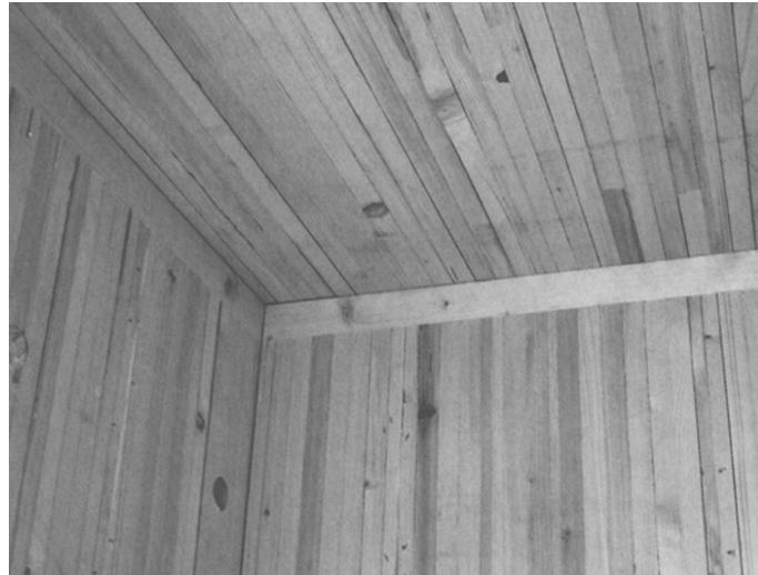
Figure 5.20: Corner detail of a stacked plank construction [21, 122]
