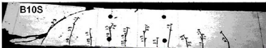
Figure 5.5 Crack pattern of beam B10S at failure
