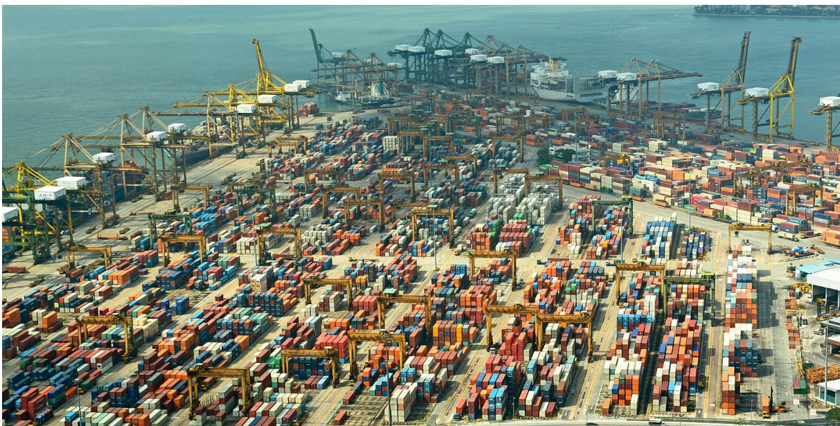
Figure 13 - Illustration of Singapore 2nd largest container terminal in the world ( Google)
