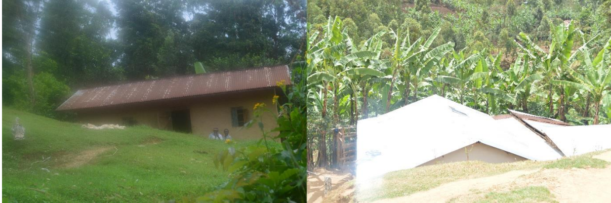
Figure 9: Houses constructed after levelling the ground leaving a hanging cliff
