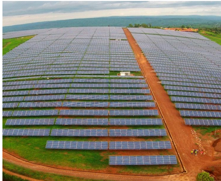
Fig. 2.8: utility-scale of 8.5MW PV power plant constructed in Agahozo-Shalom Youth Village in Rwanda [9].
