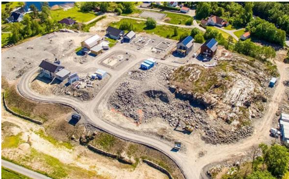
Figure 4.1 House C6 in the Skarpnes Smart house project
