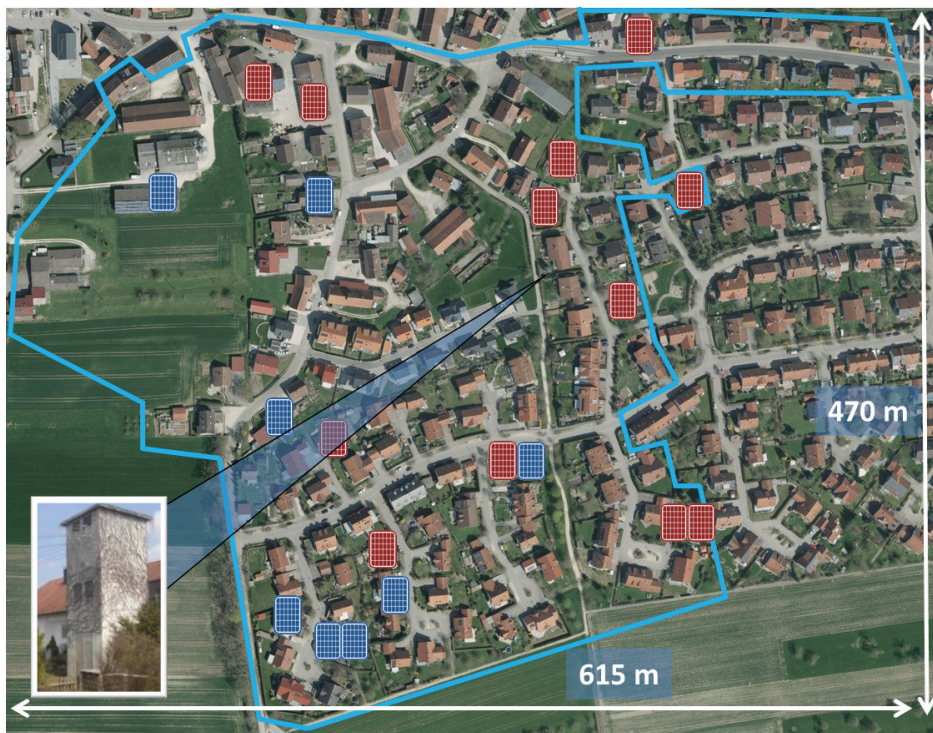
Figure 3.3: Aerial image of the test site. The border of the test site is illustrated as a blue polygon. The PV systems equipped with smart meters are marked in red, others in blue. The position of the transformer station is marked embedded image. Airborne image © City of Ulm, measurement department
