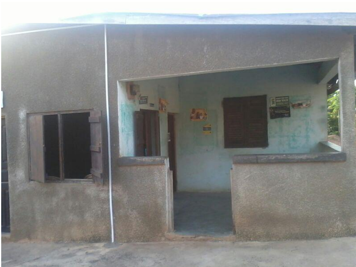
FIGURE 12: Current state of the CHPS compound in Nsanfo
