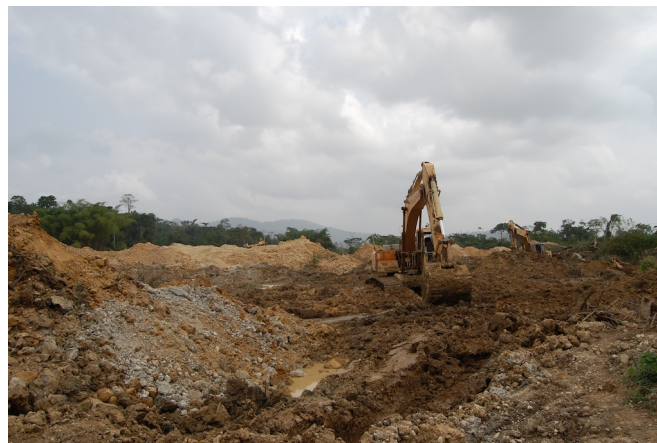
Figure 9: Excavators at Chinese galamsey site
