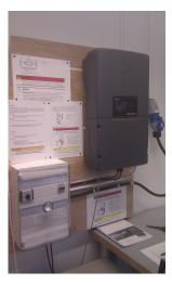
(a) Inverter and junction box installed on the plywood plate with the AC socket and user instructions.
