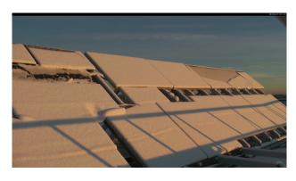
FIGURE 4.8: Partial shading from the fence on previous installed modules. Photo was taken 9:30 on January 2011 [19].
