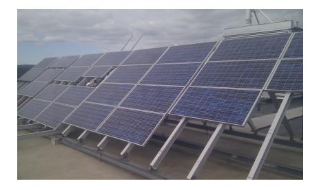
FIGURE 5.15: Configuration of the PV array after the mechanical installation.
