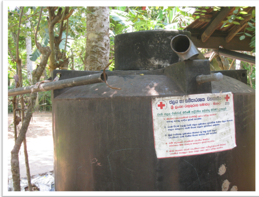
Figure 40: Photo of rainwater project in Welligama
