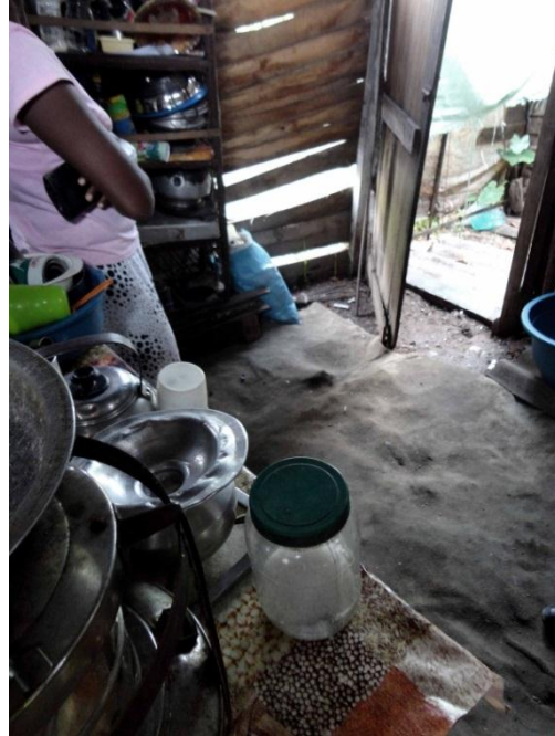
Photo B: Shack kitchen. During heavy rain and flood, water enters through the walls filling the latrine (door to the right in photo) and the kitchen. Source: Author
