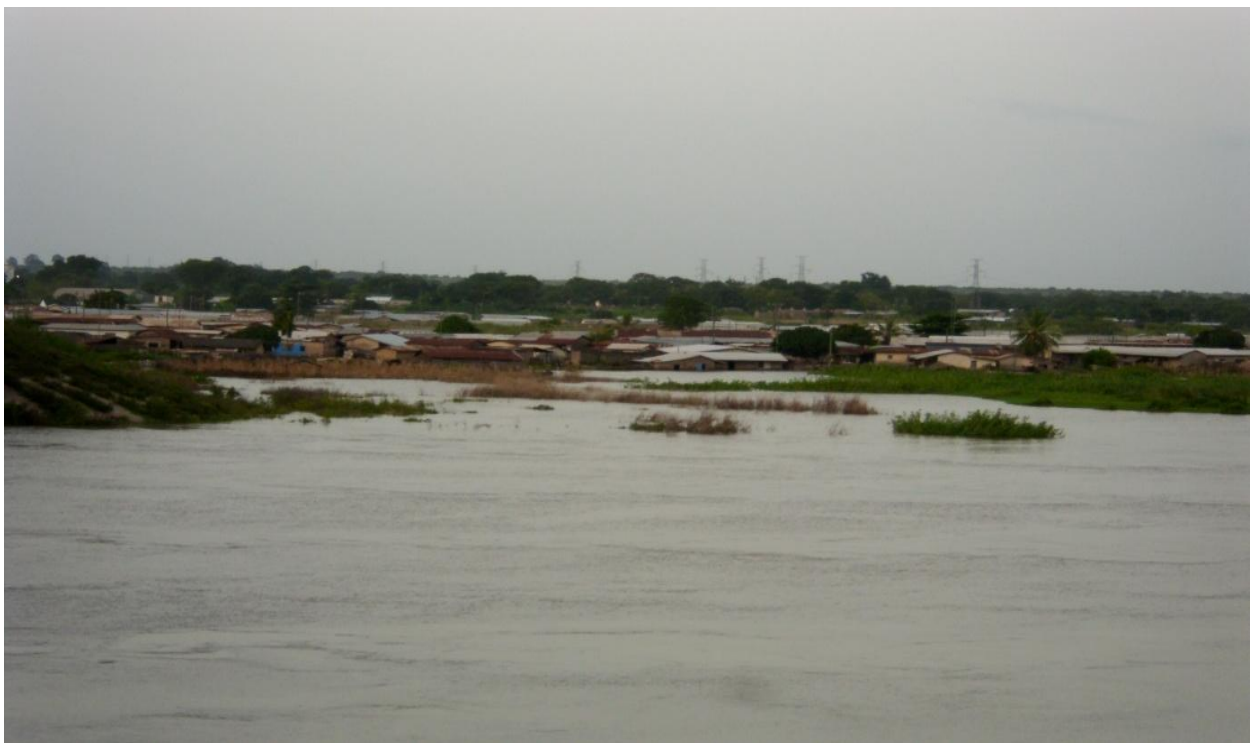
Figure 1: A Picture of a Flooded Community in Buipe But with People Still Living Close or Within the Vulnerable Areas.
