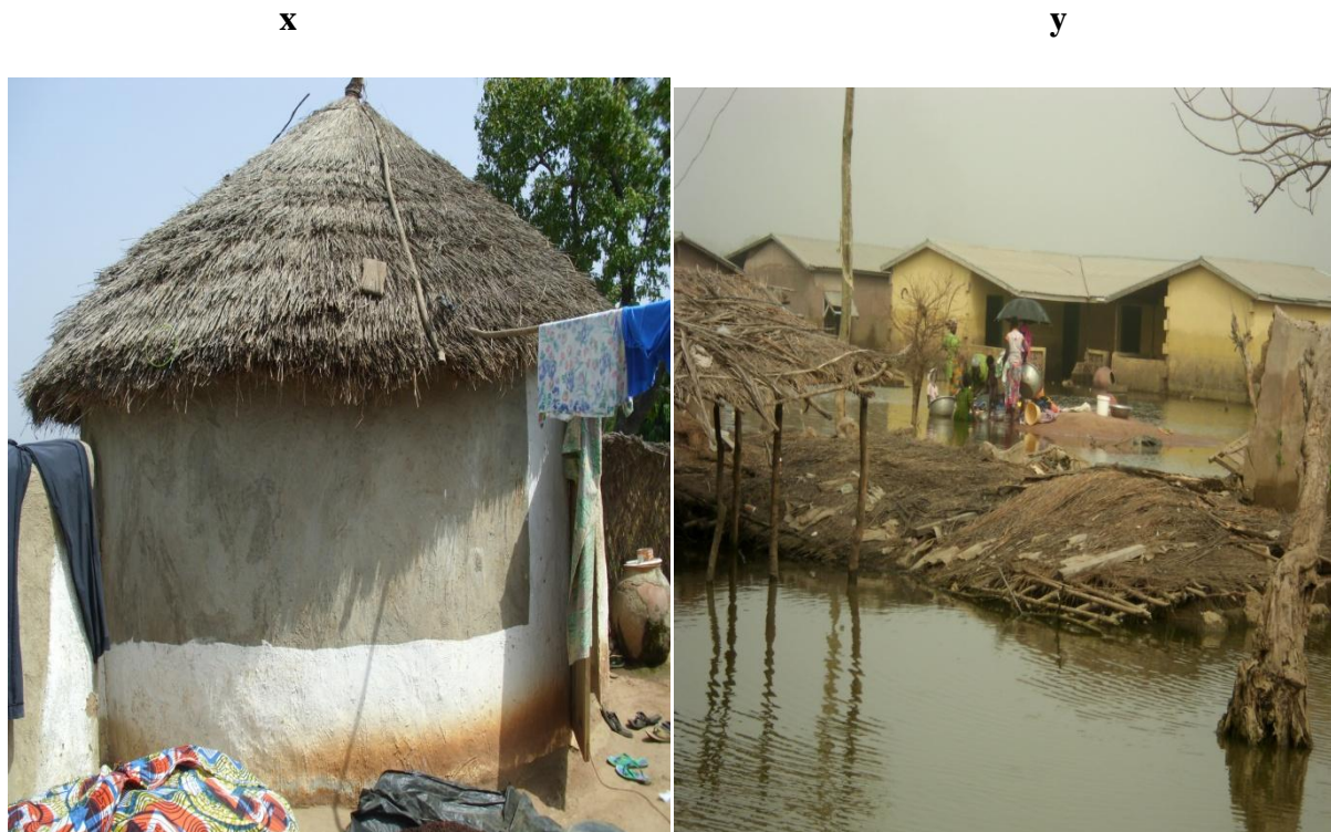
Figure 10: A Picture of A Mud House with Thatch Roof (x) and A Cement House with Aluminium Roof (y)
