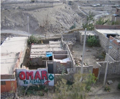
Figure 5: Next door neighbor to the CDT.
