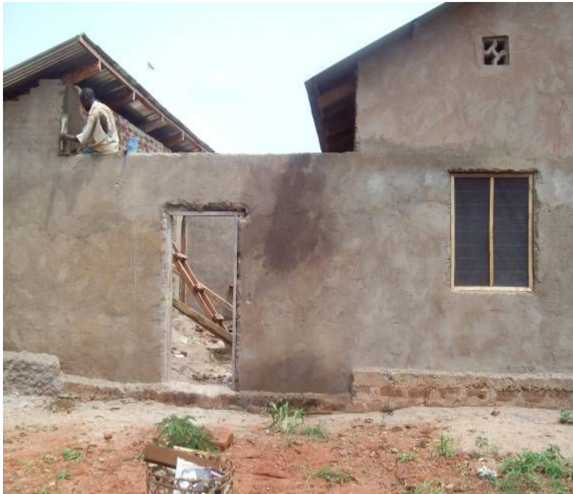
Photo 4.9: The finishing construction stage at Lugono Primary School in Mlali Ward
