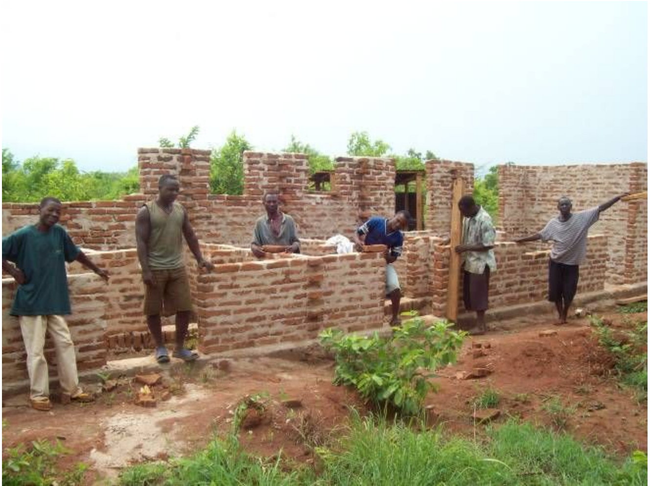
Photo 4.8: Wall construction stage at Kimambila primary school in Mzumbe Ward
