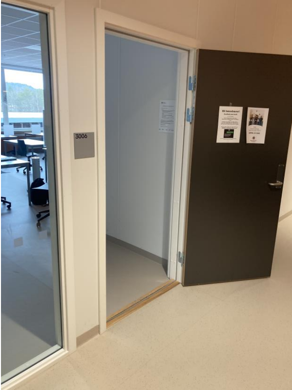
Figure 5.4 Tvedestrand Videregående Skole - Room 3006 Entrance.
