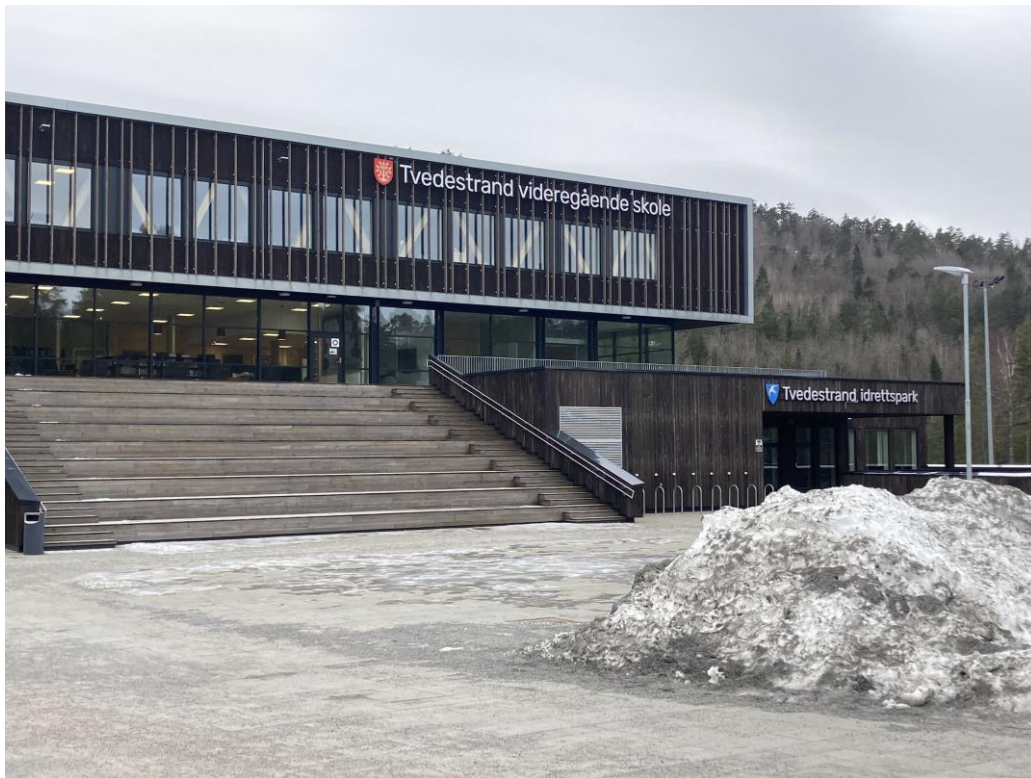
Figure 5.1 Tvedestrand Videregående Skole - Entrance.
