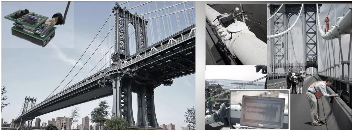
Figure 1 Structural health monitoring of a bridge [62]
