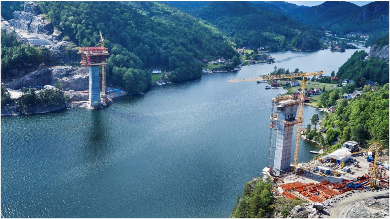
Figure 25. Aerial view of case project Mandal east-Mandal city (Google)
