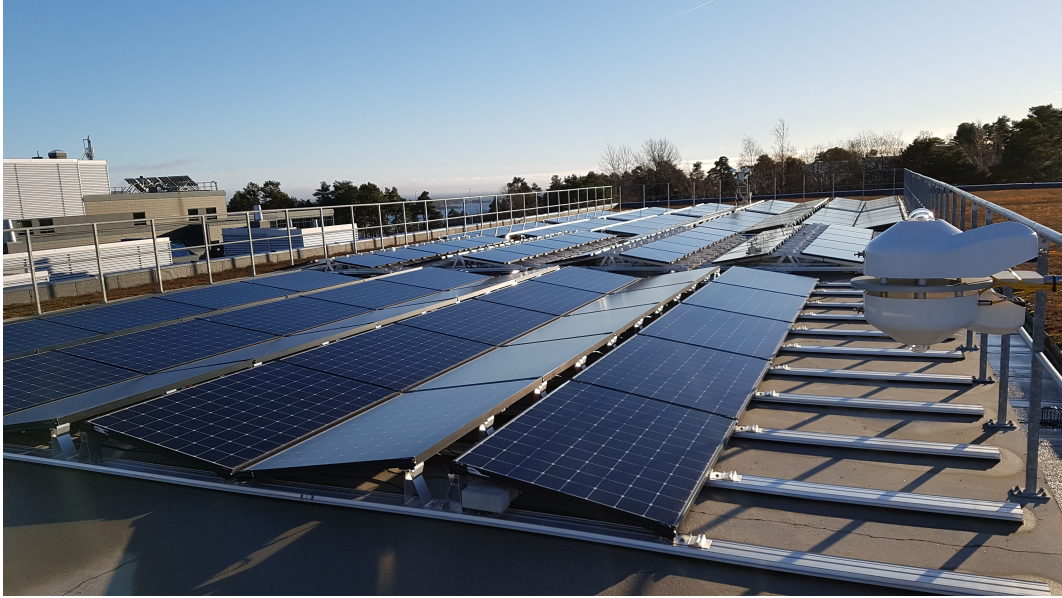
Figure 4.1: Picture of the PV modules mounted East/West with a 10^\circ angle at the roof of the University of Agder. Picture taken from North looking South.
