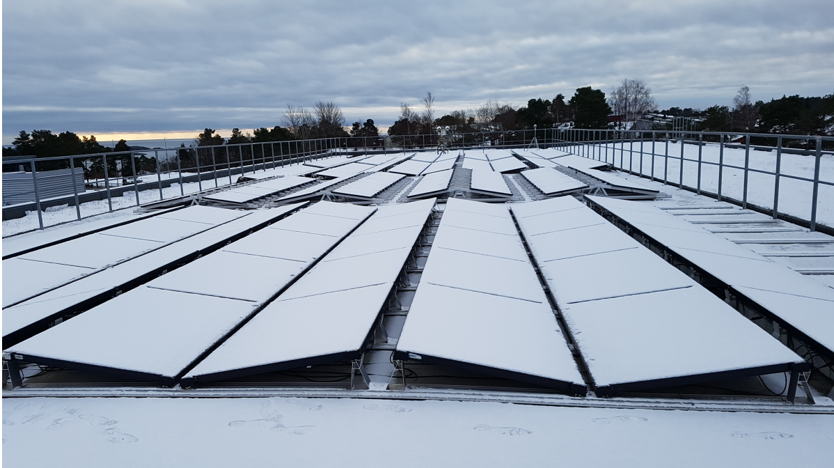
Figure A.3: Light cover of snow on the 10° modules at UiA. Picture taken in January 2021
