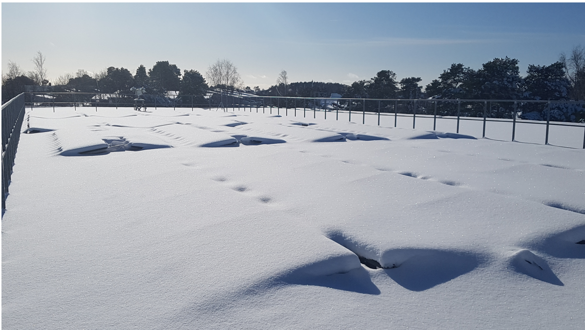
Figure A.4: Heavy cover of snow on the 10° modules in February 2020.
