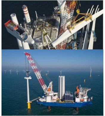
Figure 1 Examples of offshore wind turbines during installation (top: single-blade installation; bottom: nacelle installation. source: A2SEA A/S)
