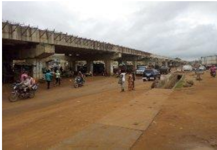
Figure 9: Showing uncompleted and abandoned flyover bridge at Akute. Source: Fieldwork (2020)
