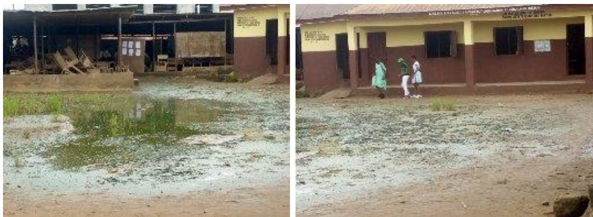
Figure 8 showing premises of the only public primary and secondary schools in Akute with pupils in background (left) taking classes in dilapidated structures and some students doing a dance rehearsal (right). Source: Fieldwork (2020)
