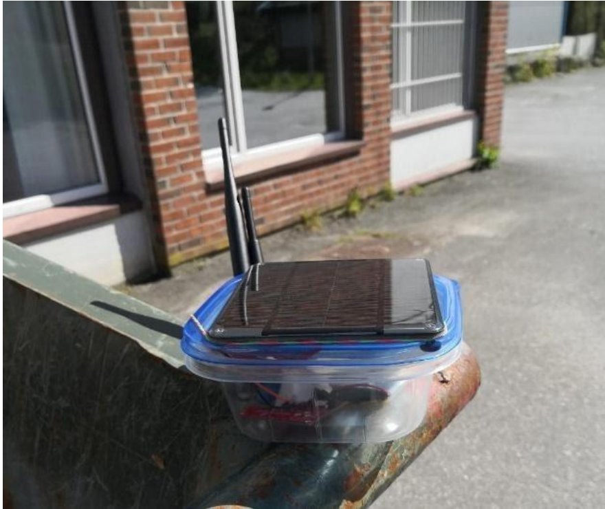
Figure 4.34: Sensor node placed on the longest distance from the sensor
