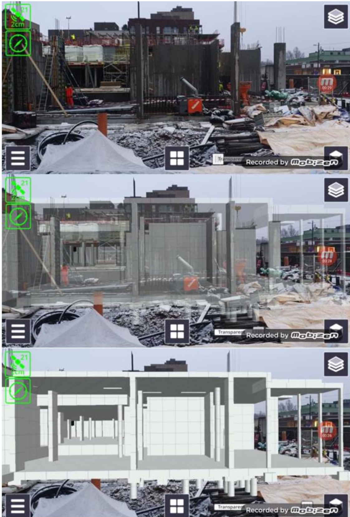
Figure 29 Future state being illustrated virtually over the real world (Appendix – D.2).
