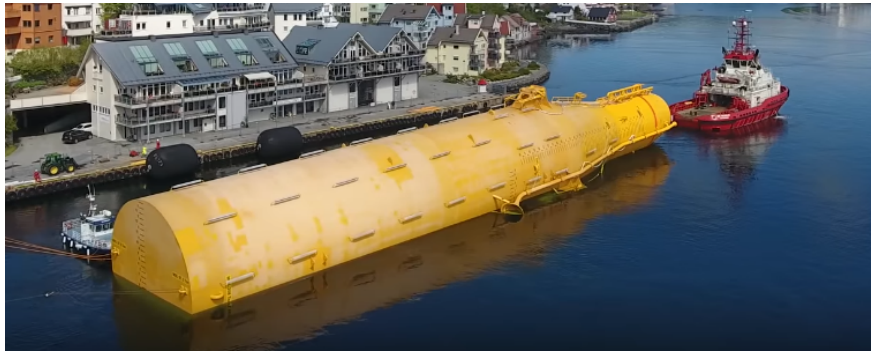
Figure 1.2: Transport of platform to deep-water area [2].
