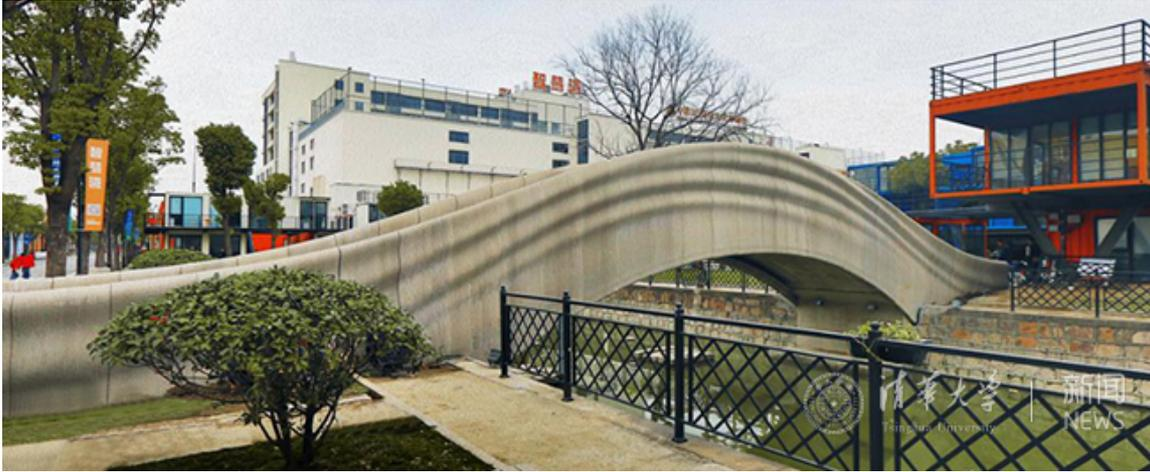
*Figure 3.7 3D printed concrete bridge in Wisdom Bay Industrial Park in China [55].*
