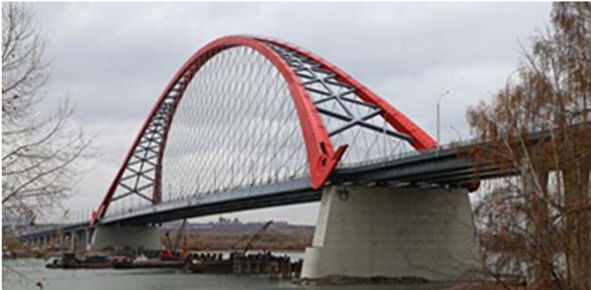
Figure 20. Network arch over Ob in Siberia. Span 380m.
