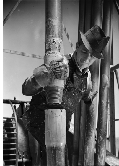
(a) Traditional roughneck connecting the box-end (lower part of the pipe joint) and the pin-end (upper part of the pipe joint).
