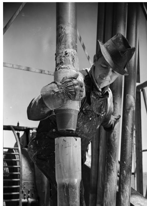
Figure 1. Old fashion roughneck connecting drill pipe. Here he is supporting the pin end tool joint to be placed in the box end of the drill pipe below. (Image, Wikimedia commons.)
