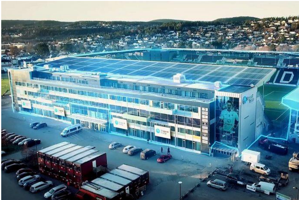
Figure 5 Skagerak Arena Football Stadium with Photovoltaic Panels and Battery Storage [55].
