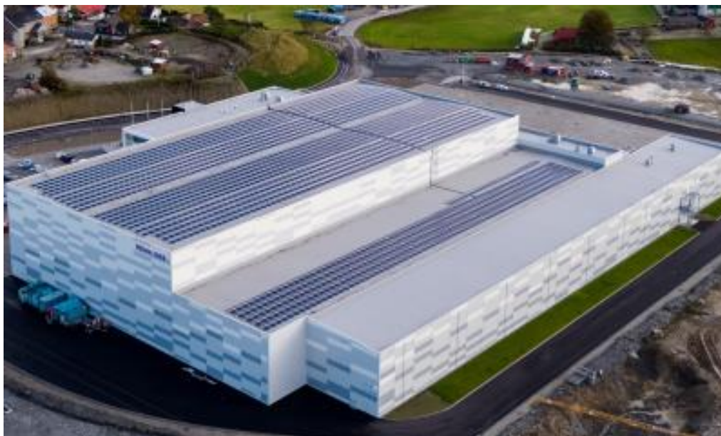
Figure 3 Grocery Distribution Central in Sandnes with Photovoltaic Installation and Battery Storage [51].
