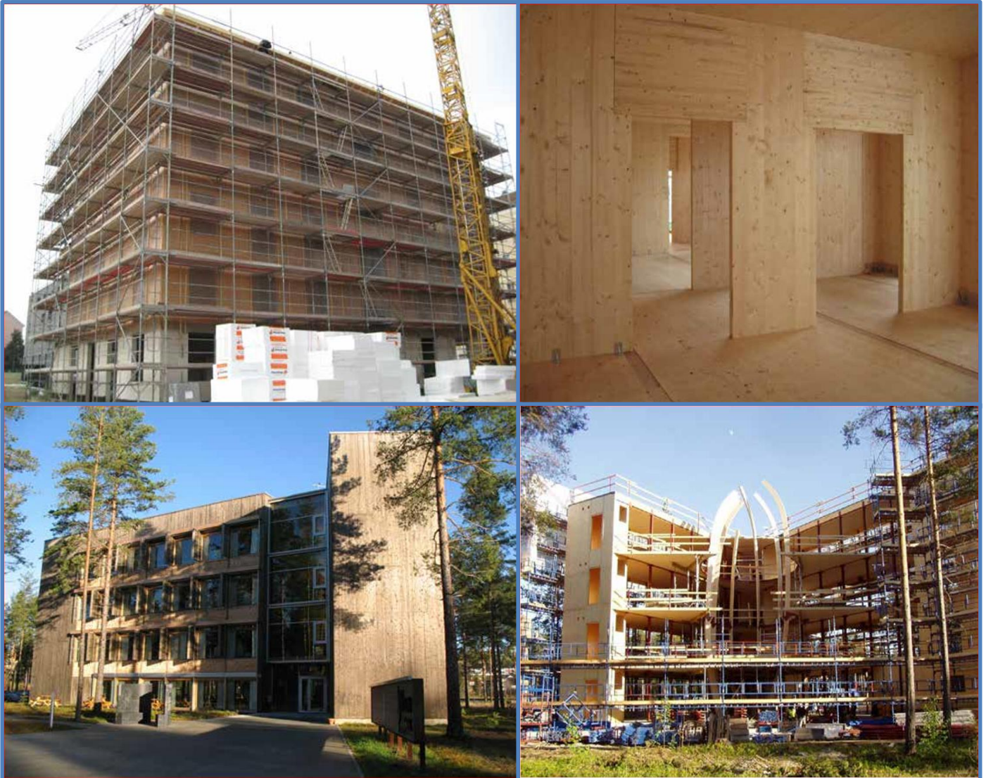
Figure 3.12: Examples for CLT constructions. Multi-family building Berlin, Germany(above). Viken skog BA, Hønefoss, Norway(down)[7]
