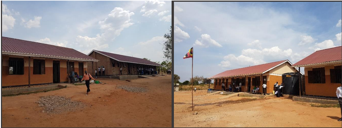
A collage showing part of the three (3) class room blocks at Rhino Camp High School. Photo: Tererai Obey Sithole (2018).
