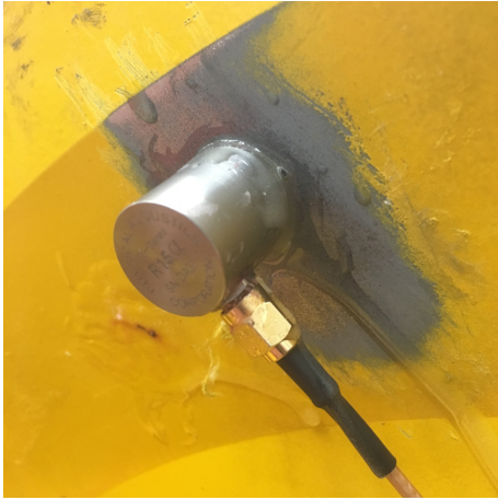
(a) The paint of the sheave is removed as it's believed to dampen AE signals
